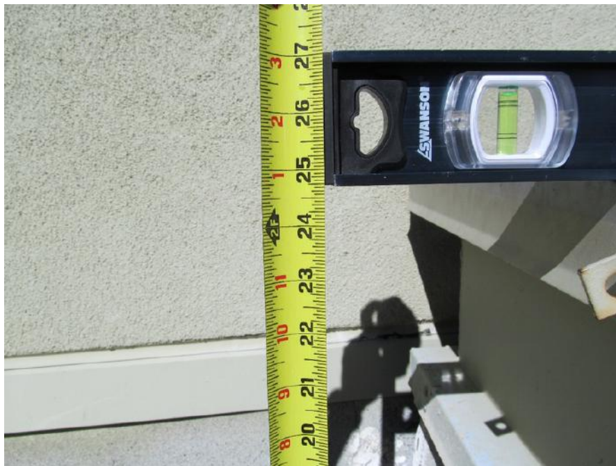
PK-01.087; 11/04/2014; Building 6; Roof; The cap sheet is \pm 24 \frac{3}{4} " from the roof hatch level \pm 6 " from the edge over the latching mechanism / receiving bolt.
