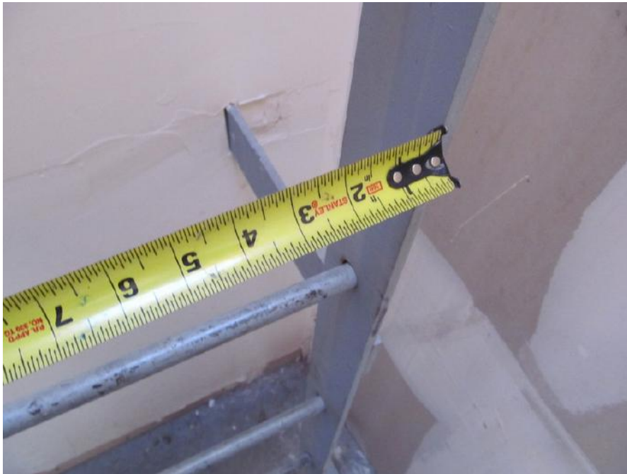
PK-01.061; 11/04/2014; Building 6; Roof Access; Step ladder inside dimension is \pm 15 \frac{7}{8} ".
