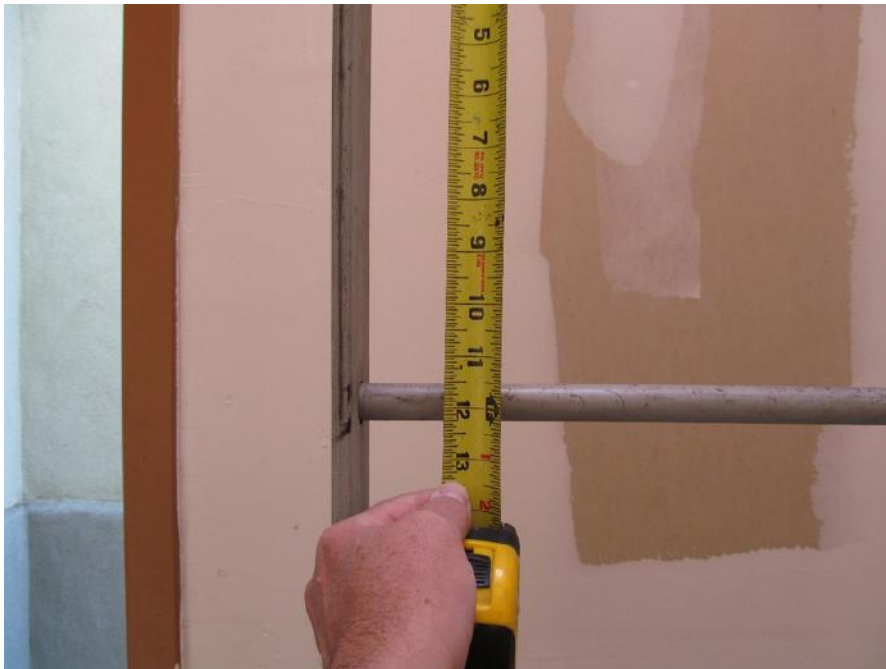
PK-01.110; 11/04/2014; Building 6; Roof Access; Step ladder rings at 12" on center.
