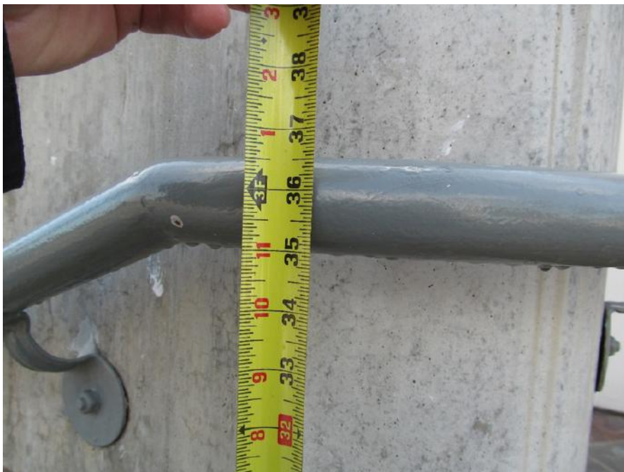
PK-01.100; 12/17/2014; Stairway; East riser section with handrail \pm 36 \frac{1}{2} " above top of nosing.
