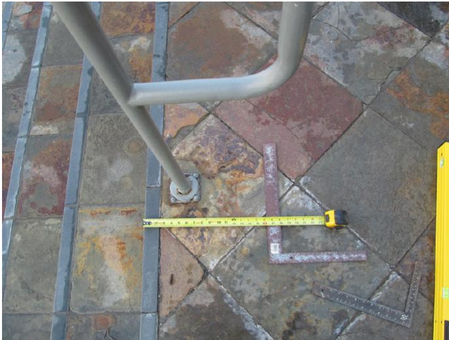
PK-01.053; 12/17/2014; Stairway; Stairway extension is +/- 17 15/16". See A/3 at top.
