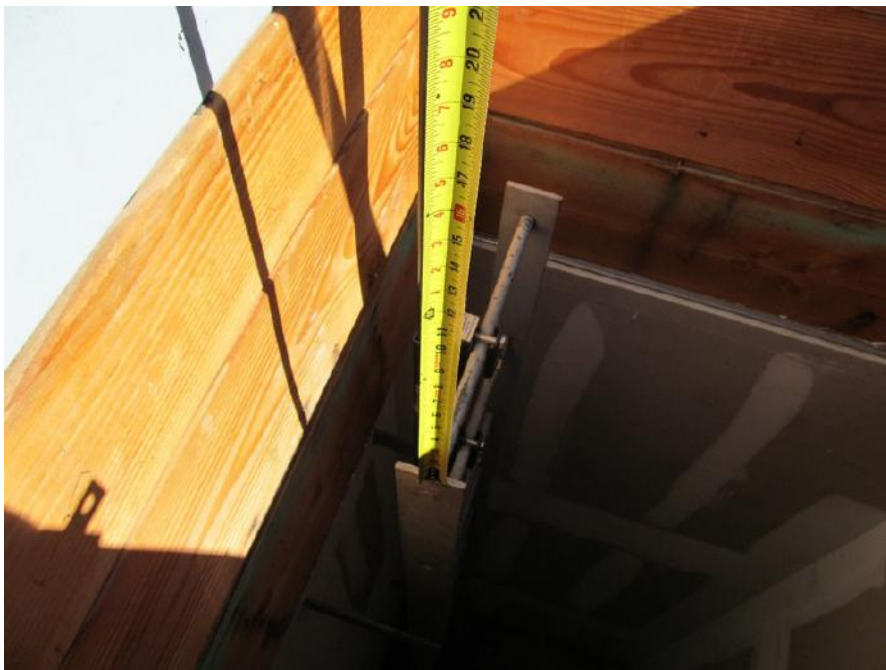
PK-01.076; 11/04/2014; Building 6; Roof Access; Top of the step ladder handrail to the roof hatch is \pm 27 \frac{5}{8} ".
