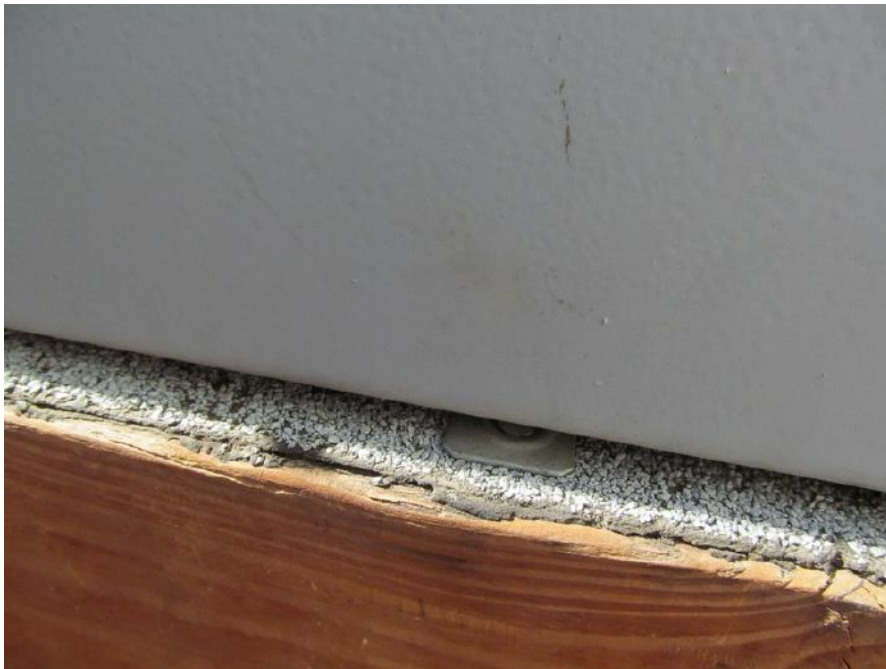
PK-01.045; 11/04/2014; Building 6; Roof Access; Roof hatch curb with built up roof cap sheet and disc nails visible along top edge beneath the roof hatch metal flange / flashing.
