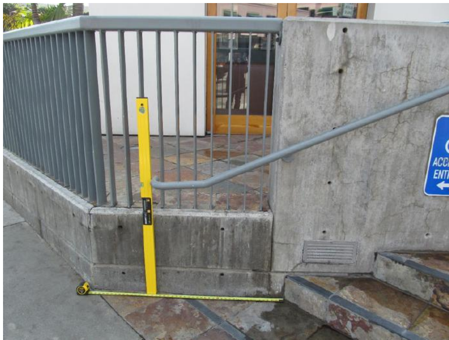
PK-01.104; 12/17/2014; Stairway; East riser section with handrail +/- 34 1/2" above the bottom nosing with +/- 31" extension.
