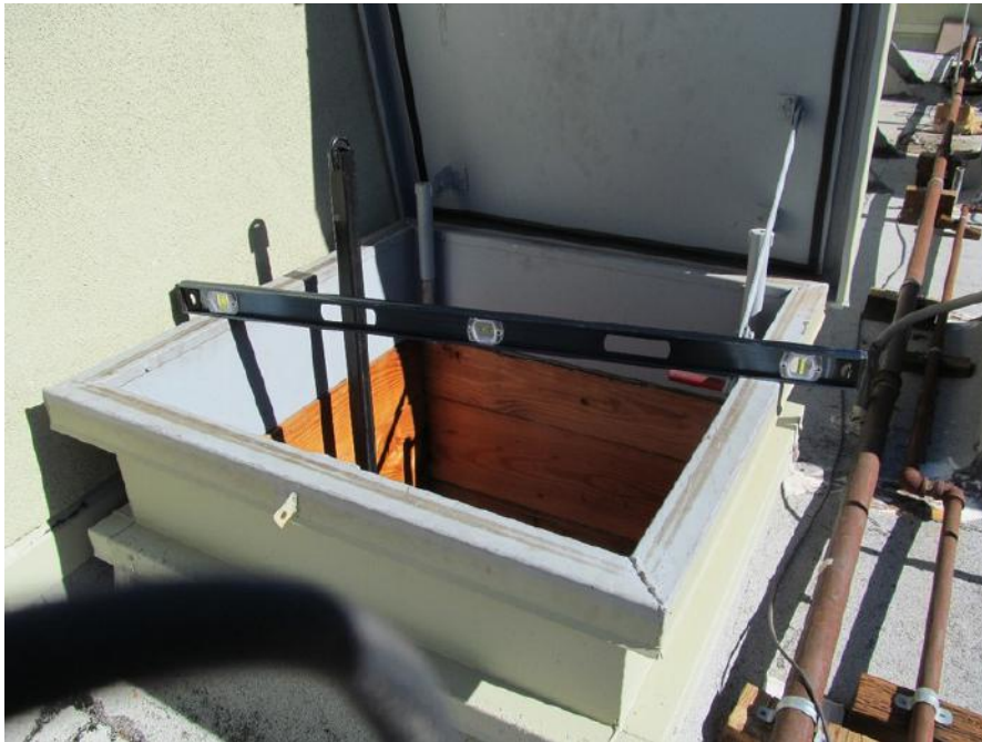
PK-01.016; 11/04/2014; Building 6; Roof; Top edge of the roof hatch is 13 -15 3/4" from the slab on grade concrete floor below. See A/2.
