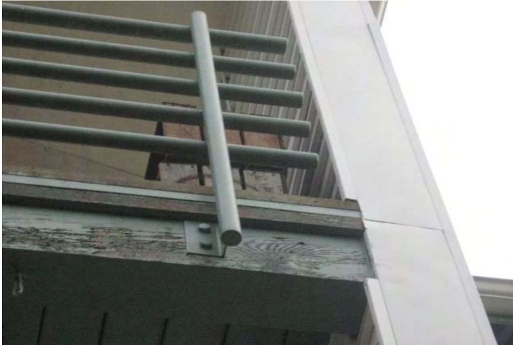
SM 01.038 Unit #49; Back elevation; Deck. Main guardrail fastened to beam with large lag bolts.
