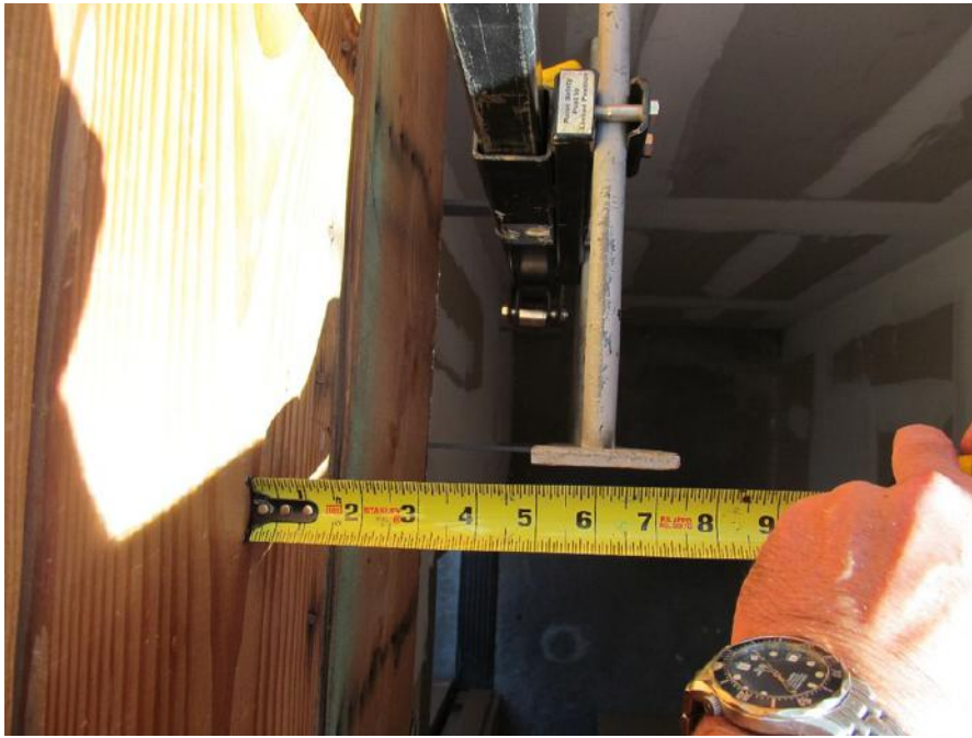
PK-01.108; 11/04/2014; Building 6; Roof; 13 " wide step ladder side rail is 4 3/4" from the well framing.
