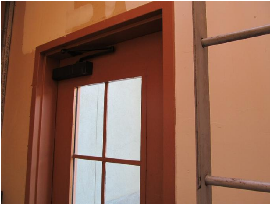
PK-01.127; 11/04/2014; Building 6; Roof Access; Roof access door jamb is \pm 32 \frac{1}{2} " from wall. Window opening is \pm 40 " away from wall.
