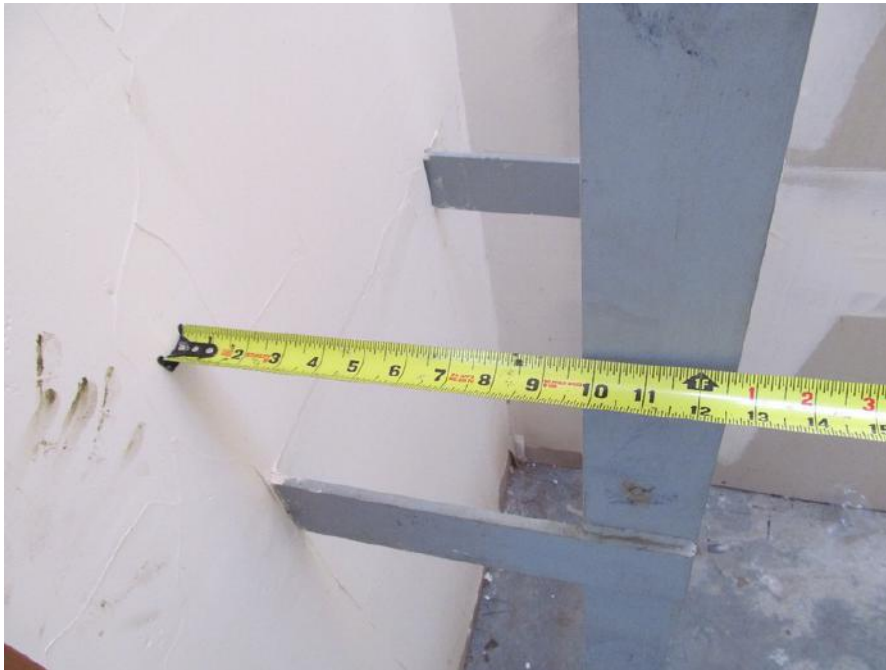
PK-01.111; 11/04/2014; Building 6; Roof Access; Step ladder is \pm 9 \frac{3}{4} " from gypsum wallboard wall.
