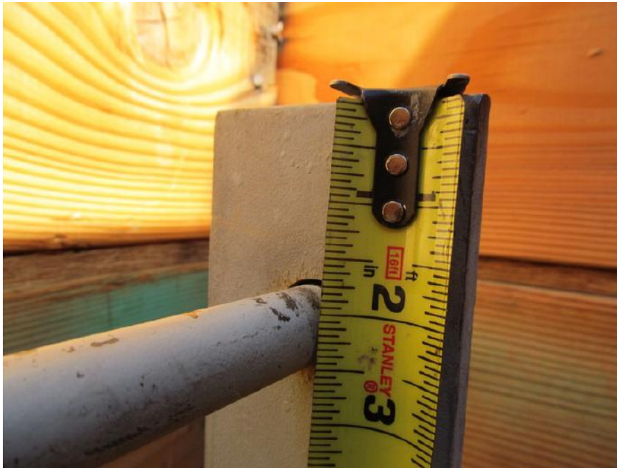
PK-01.123; 11/04/2014; Building 6; Roof Access; Top ring \pm 1 \frac{3}{4} " below top of side rail.
