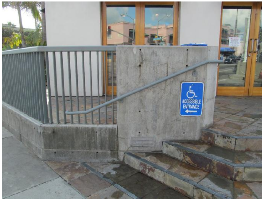
PK-01.101; 12/17/2014; Stairway; East riser section with handrail +/- 34 1/2" above the bottom nosing with +/- 31" extension.
