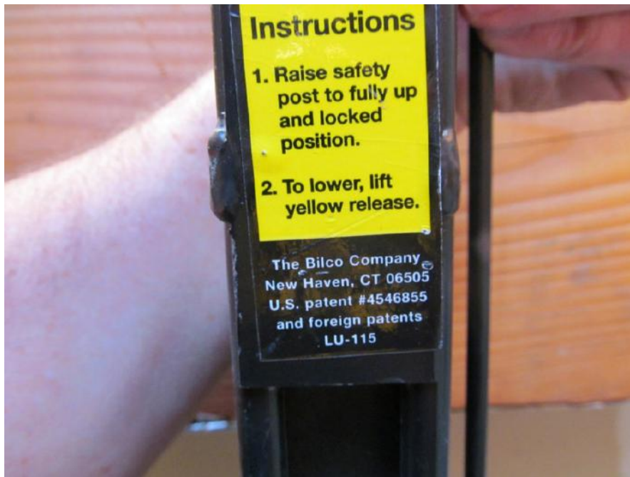
PK-01.125; 11/04/2014; Building 6; Roof Access; Safety post. LV-115.
