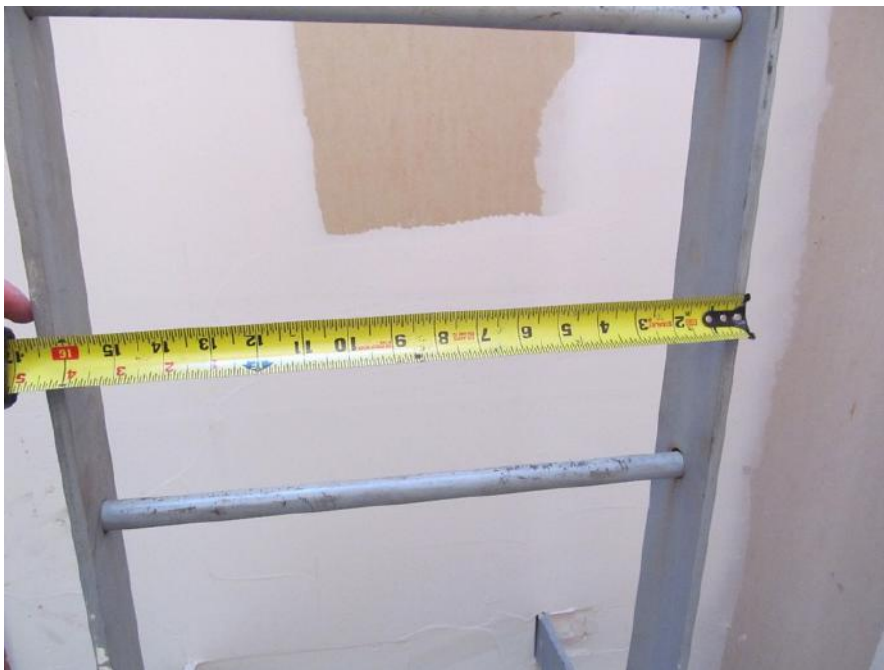
PK-01.059; 11/04/2014; Building 6; Roof Access; Step ladder outside dimension is \pm 16 \frac{1}{2} ".
