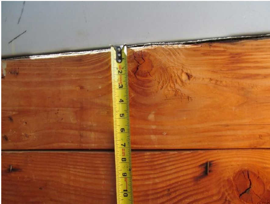
PK-01.036; 11/04/2014; Building 6; Roof Access; Curb \pm 7" deep. See A/2.
