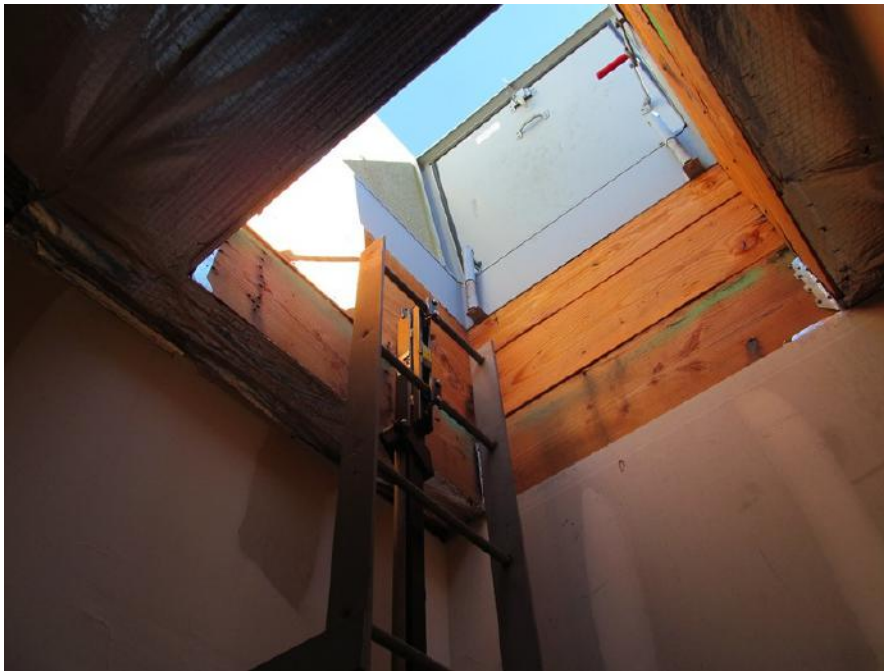
PK-01.006; 11/04/2014; Building 6; Roof Access; Step ladder approach to roof hatch.
