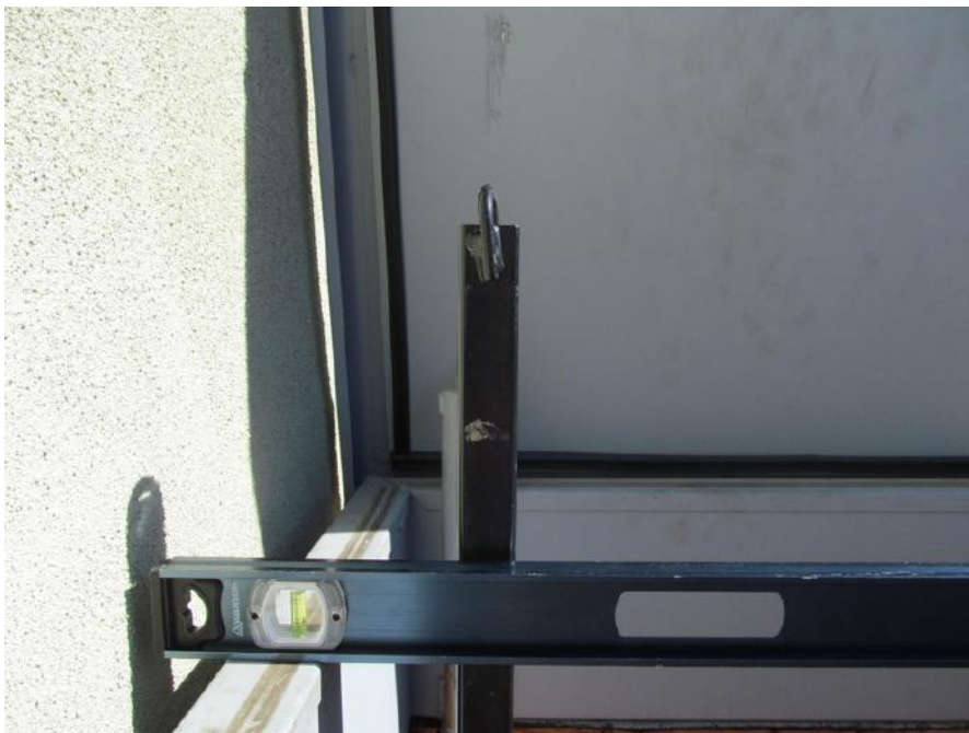
PK-01.019; 11/04/2014; Building 6; Roof; Top of safety pole extends 8 1/2" above the top edge of the roof hatch.
