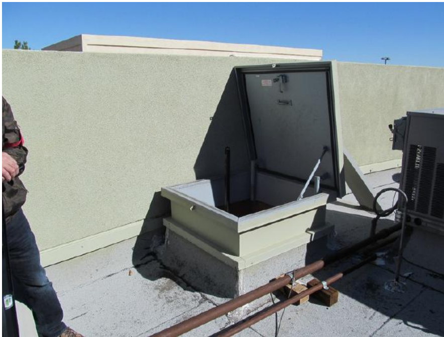
PK-01.013; 11/04/2014; Building 6; Roof; Roof hatch open position from the roof side ± 13' - 5 3/4" from top of hatch to the slab on grade below.
