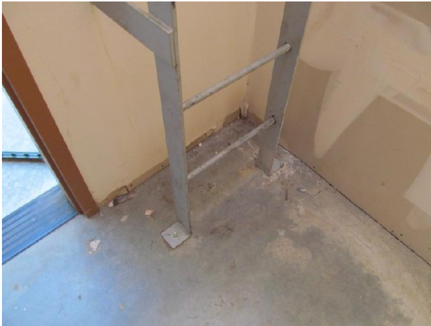
PK-01.055; 11/04/2014; Building 6; Roof Access; Bottom of the step ladder with 3" square plates for attachment at slab on grade concrete with wall attachments with walls taped and molded, no texture.
