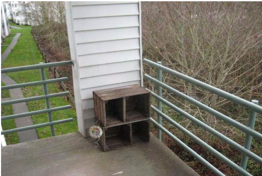
SM 01.043 Unit #49; Back elevation; Deck railing. Side guardrail at left, main guardrail at right. Note attachment to wall at right side of left guardrail.
