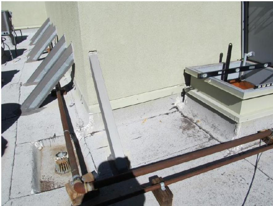
PK-01.094; 11/04/2014; Building 6; Roof; Parapet wall, knee brace is \pm 46 \frac{1}{2} " from the hatch opening.
