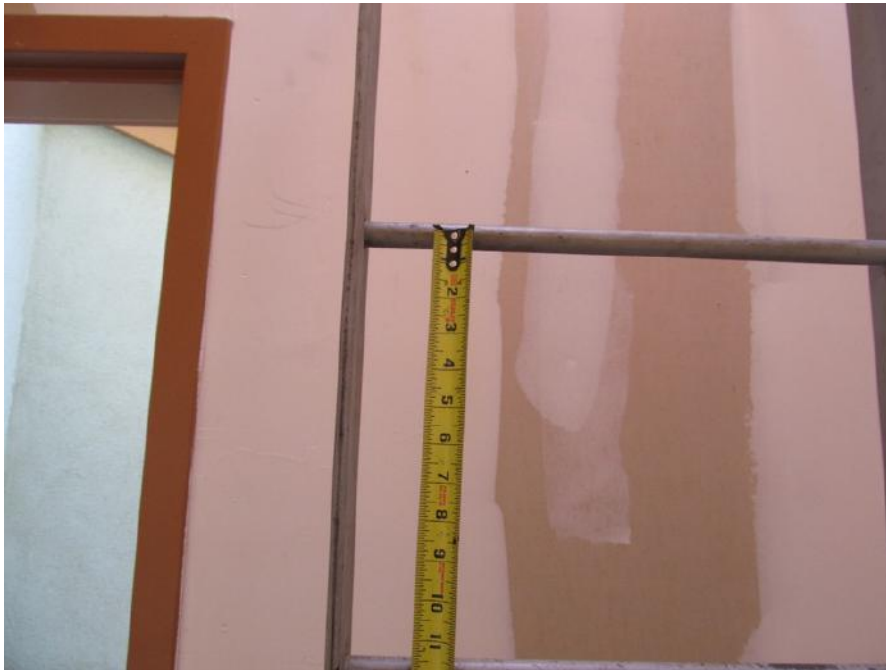
PK-01.109; 11/04/2014; Building 6; Roof Access; Step ladder rings at 12" on center.
