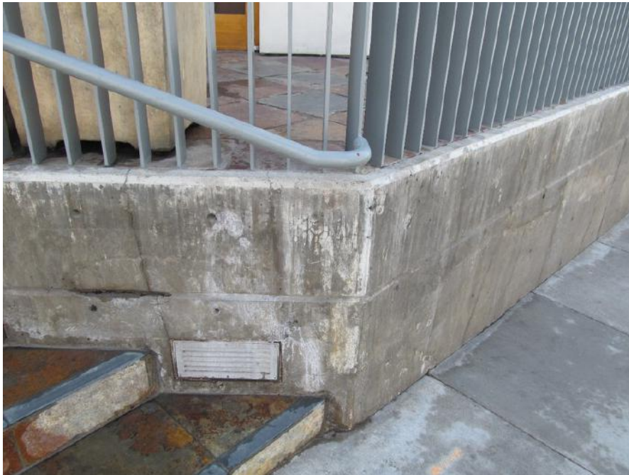
PK-01.094; 12/17/2014; Stairway; West riser section bottom of handrail extension \pm 2 \frac{3}{4} " beyond last riser, handrail is \pm 33 \frac{15}{16} " above the last nosing.
