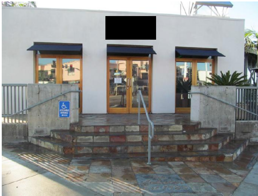
PK-01.029; 12/17/2014; Stairway; Front elevation of stairway looking South, fan shaped stairway with middle section of stairway with 4 risers with bisecting handrail and 2 angled stairway to the East and West. Right hand side (west side) with 5 risers to sloping pathway. Left hand side (east) parallel to Colorado with 3 risers, level with Colorado.
