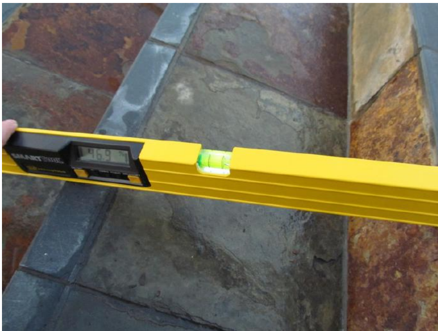
PK-01.068; 12/17/2014; Stairway; West risers with 46.4% range between nosing. Quick check west risers 46.7% range between risers.
