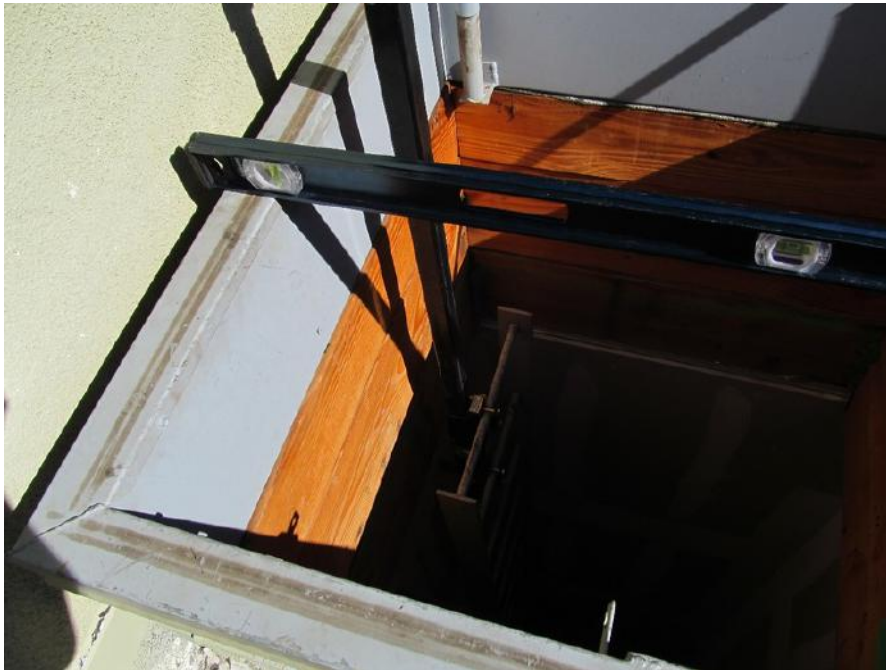
PK-01.075; 11/04/2014; Building 6; Roof Access; Top of the step ladder handrail to the roof hatch is \pm 27 \frac{5}{8} ".
