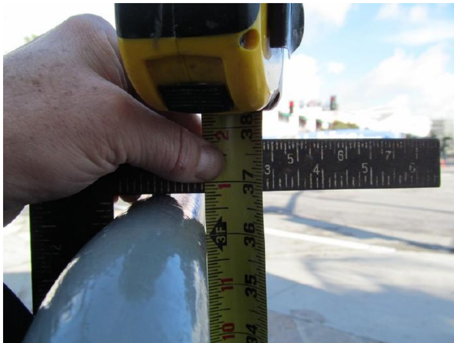
PK-01.049; 12/17/2014; Stairway; Middle section top is +/- 36 13/16" above finished floor at top.
