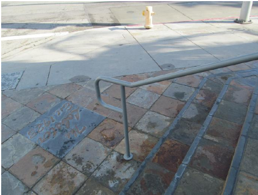
PK-01.054; 12/17/2014; Stairway; Stairway extension is +/- 17 15/16". See A/3 at top.
