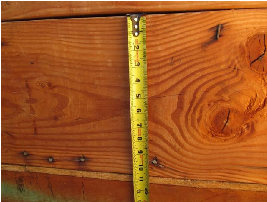
PK-01.033; 11/04/2014; Building 6; Roof Access; Depth of the hip strip blocking \pm 11 " thick. See A/2.
