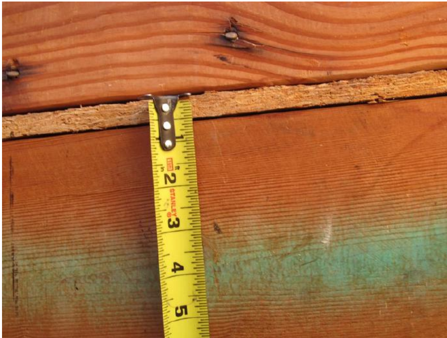
PK-01.032; 11/04/2014; Building 6; Roof Access; Structural sheathing \pm 1/2 " thick. See A/2.
