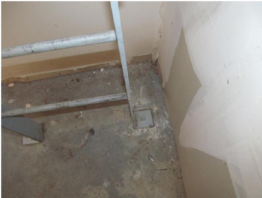
PK-01.073; 11/04/2014; Building 6; Roof Access; Step ladder with texture over the 3" square plates at the horizontal attachments side grab.
