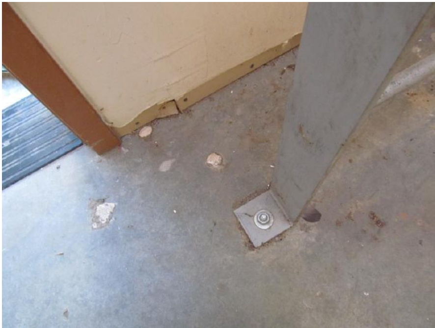
PK-01.113; 11/04/2014; Building 6; Roof Access; Bottom 3" square plates. No signs of pilot / drill holes in slab on grade.
