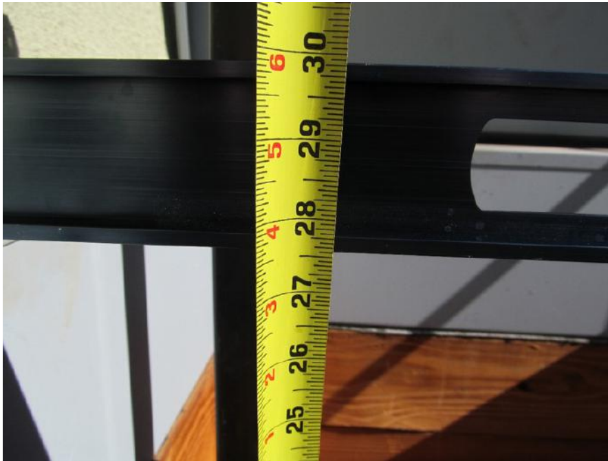
PK-01.077; 11/04/2014; Building 6; Roof Access; Top of the step ladder handrail to the roof hatch is \pm 27 \frac{5}{8} ".
