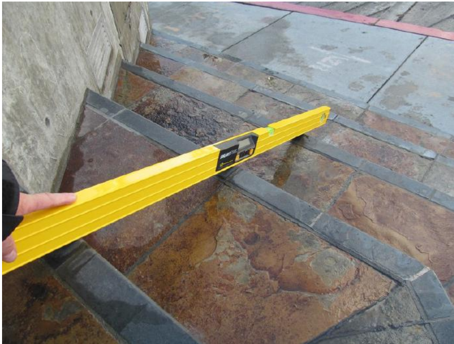
PK-01.063; 12/17/2014; Stairway; West risers with 46.4% range between nosing. Quick check west risers 46.7% range between risers.
