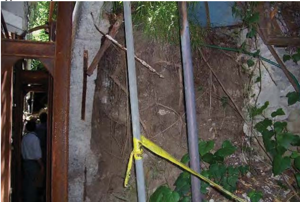
Right elevation; overview of end of wall - note separate vertical stages. Lower wall CIP against soil (+/- 5'6"). Cold joint at 4'6".
