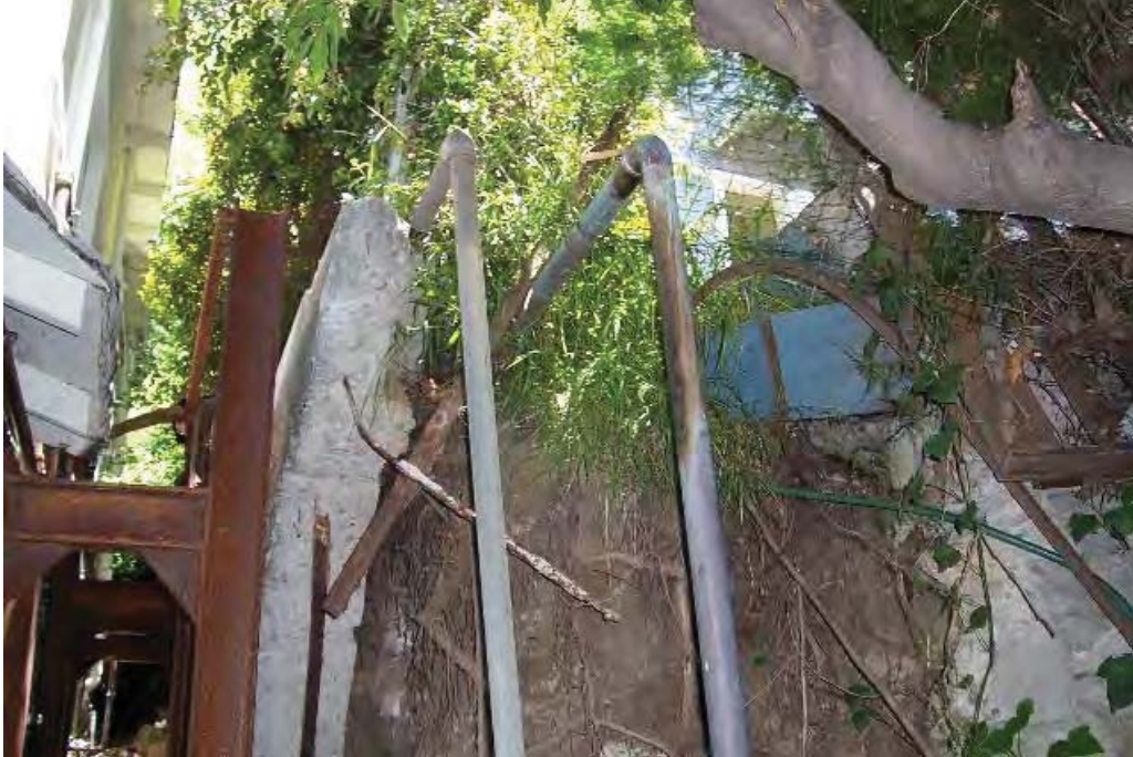
Front/right elevation; area at end of failure wall - temporary shoring - unreinforced CIP wall, plant material in exposed soil. Second unreinforced "rubble" retaining wall to right, approximately 4 - 5' tall.
