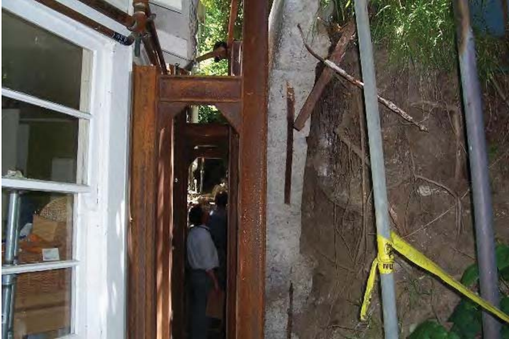
Right elevation; upper wall, temporary shoring frame.
