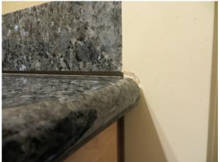
AP-02.175; Bath #2; Significant movement of Bathroom is located in the proximity of the entry.
