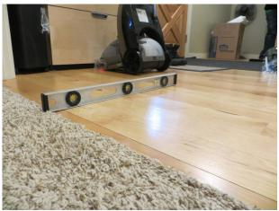
AP-02.089; Entry; High point, linear (similar to same condition in kitchen). Floor levelness does not conform to industry standards. High point is linear from entry to main living area. Separation noted at wood floors, between planks.
