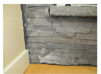
AP-02.040; Living Room; Excessive settlement of fireplace surround / cracks through masonry veneer fireplace surround / cracks through masonry surround
