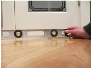
AP-02.071; Kitchen; High spot noted at pantry, and AP-02.072; Kitchen continuous from pantry to across kitchen towards refrigerator. High spot is very linear. Floor levelness out of industry tolerances. Slight separation (gaps) at wood flooring.
