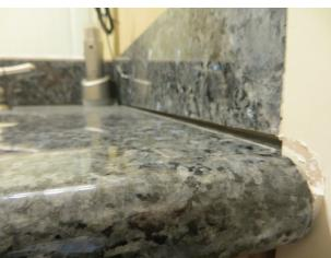
AP-02.173; Bath #2; Excessive settlement at countertop backsplash interface with horizontal surface / missing and voids at sealants
