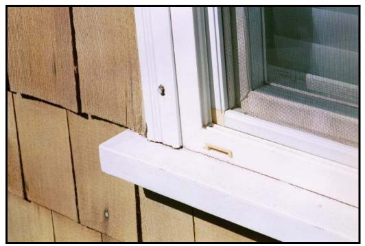
PF 03-12-060 jpg Window casing with popping nail and separation at sill.
