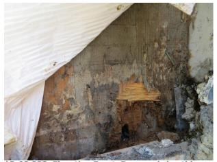
AP-02.233; Elevation Front; Damaged sheathing behind masonry veneer / previous water intrusion, not current. Masonry veneer over lath over WRB system.
