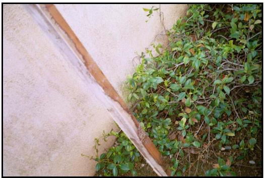
PF 09-16 088 .jpg Wood (Douglas Fir) from exterior window sill. All surfaces not primed before installation.
