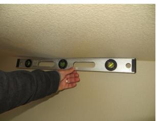
AP-02.112; Office; Office ceiling uneven, exceeding AP-02.185; Stairs to Upstairs; Uneven / bowed industry standards and tolerances. Cabinets noted towall at entry stairs to upstairs. be level.
