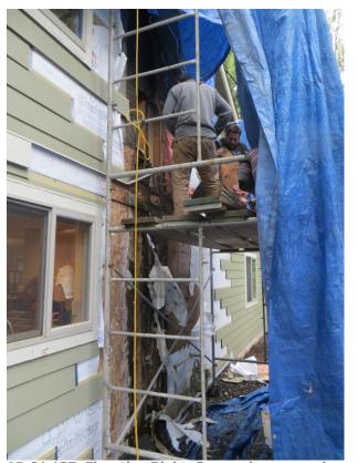
AP-01.137; Elevation Right; Severe damage and active water intrusion event. Source of water intrusion at roof-to-wall interface / lack of diverter flashings / failed condition at roof assembly / failed condition at siding components.
