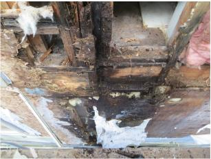
AP-01.138; Elevation Right; Active water intrusion event at right elevation of structure. Damaged framing / structural analysis required.
