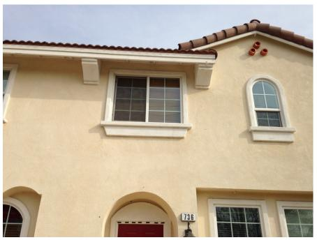
PV-01.100; 12/11/2014; B7/736; Elevation Front; Valley drains over entry door
