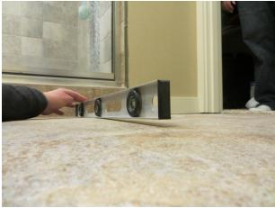
AP-02.136; Master Bath; Excessive movement and settlement at master bath tile floor
