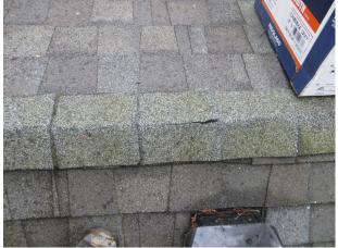
AP-02.317; Roof; Damaged shingles at ridge.
