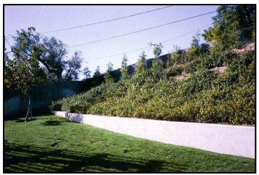
MP 01.27 027 jpg Rear yard retaining wall. One area drain behind wall at orange tape measure.
