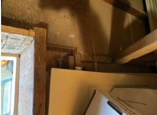
AP-02.290; Attic; Altered bottom chord of truss / missing bottom chord.
