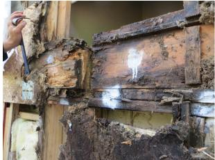
AP-02.214; Elevation Right; Severe damage at rim joist.
