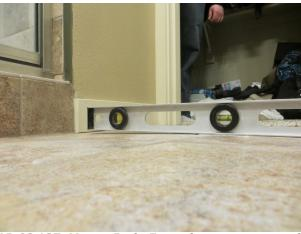
AP-02.137; Master Bath; Excessive movement and settlement at master bath tile floor
