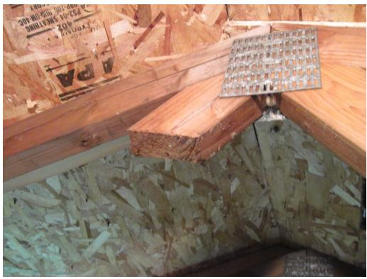
Photograph 10: Attic truss with web members removed
