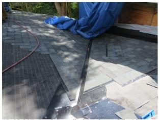
AP-02.397; Roof; Installation of metal flashing components / ongoing repairs.
