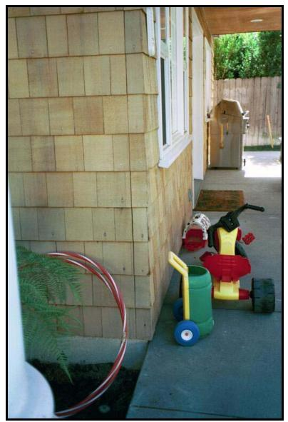
PF 02-21-045 jpg Line of siding at corner has a separation. Typical throughout.
