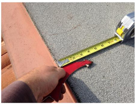
PV-01.172; 12/11/2014; B5; Roof; Membrane not sealed at drip edge
