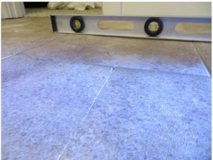
AP-02.143; Master Bath; Cracked / inadequate support for floor tile assembly / settlement
