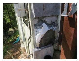
AP-02.207; Elevation Front; Garage left portal, removal of masonry at base of wall / interface to concrete footing.
