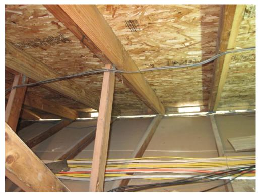
Photograph 9: Garage attic truss web members removed
