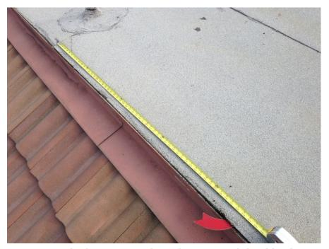
PV-01.143; 12/11/2014; B4; Roof; Membrane not sealed at drip edge
