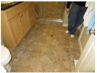
AP-02.134; Master Bath; Excessive movement and settlement at master bath tile floor
