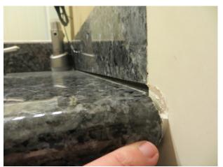
AP-02.174; Bath #2; Significant movement of granite counter-top at upstairs bathroom. Bathroom granite counter-top at upstairs bathroom. is located in the proximity of the entry.
