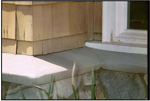
PF 01-10-010 jpg Formed concrete cap between siding and veneer below buries window trim at sill.
