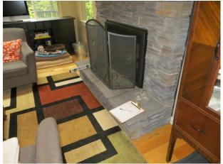
AP-02.035; Living Room; Excessive settlement of fireplace surround / cracks through masonry veneer fireplace surround / cracks through masonry surround
