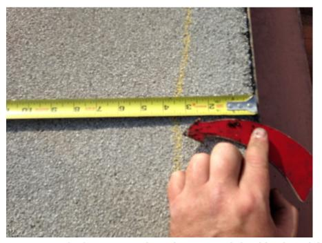
PV-01.187; 12/11/2014; B5; Roof; Membrane not sealed to drip edge at left
