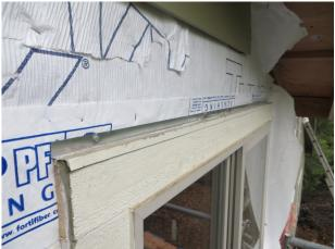
AP-01.143; Elevation Right; Improper integration of AP-02.199; Elevation Right; Improper integration of metal flashing components / Fiber cement siding sealed to metal flashing / No weep provisions
