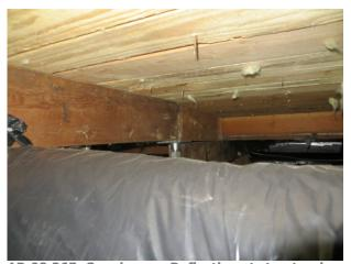
AP-02.090; Entry; High point, linear (similar to same AP-02.265; Crawlspace; Deflection at structural condition in kitchen). Floor levelness does not conform to industry standards. High point is linear from entry to main living area. Separation noted at wood floors, between planks.
