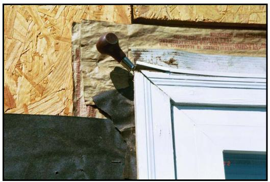
PV 03-17-155 jpg. Open joint at wood trim allows unimpeded awl penetration.
