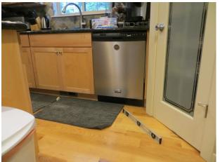
AP-02.069; Kitchen; High spot noted at pantry, and AP-02.070; Kitchen; High spot noted at pantry, continuous from pantry to across kitchen towards refrigerator. High spot is very linear. Floor levelness towards refrigerator. High spot is very linear. Floor out of industry tolerances. Slight separation (gaps) levelness out of industry tolerances. Slight at wood flooring.
