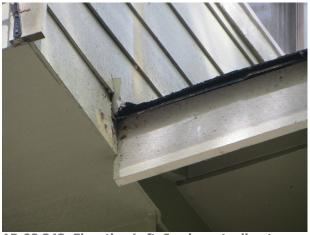
AP-02.343; Elevation Left; Inadequate diverter flashing components (typical).
