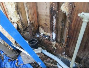
AP-02.217; Elevation Right; Severe damage at base of wall / bottom plate.
