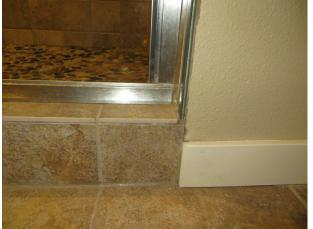
AP-02.153; Master Bath; Water reported leaking at AP-02.154; Master Bath; Water reported leaking shower enclosure frame to tile interface / inadequate sealant application and bottom of shower frame installation
