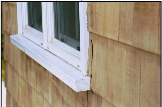
PF 10-03-03 jpg Siding is cracked and separating from window trim. Head flashing short at master bedroom – closet window.
