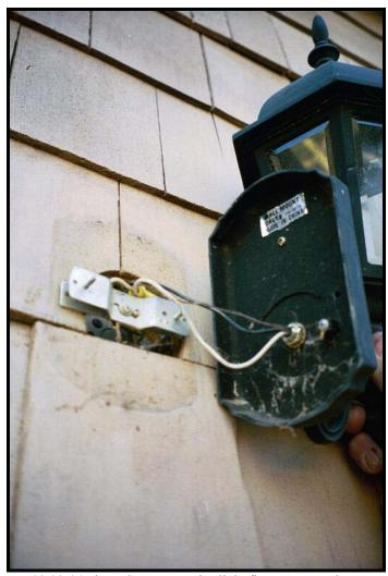
MP 02.09-045 jpg Garage exterior light fixture. No gasket or sealant. Typical all four.
