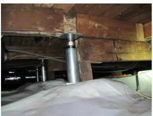
Miller Consulting Engineers-033; Uneven floor support beams. Floor jacks creating uplift, transferring through structure.
