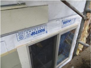
AP-02.191; Elevation Right; Improper head flashing AP-02.194; Elevation Right; Improper head integration at window head (typical).
