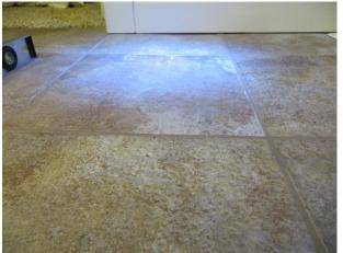
AP-02.141; Master Bath; Cracked / inadequate support for floor tile assembly / settlement
