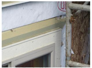
AP-01.116; Elevation Right; Improper z-metal integration at head of window (typical).
