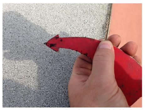
PV-01.119; 12/11/2014; B4; Roof; Membrane not sealed the drip edge
