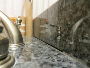
AP-02.171; Bath #2; Excessive settlement at countertop backsplash interface with horizontal surface / missing and voids at sealants
