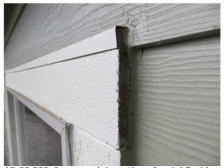
AP-02.308; Improper integration of metal flashing components / Fiber cement siding sealed to metal flashing / No weep provisions / Reverse sloped metal flashing / Un-primed end cuts
