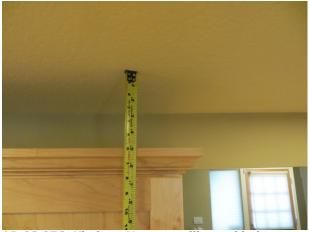
AP-02.076; Kitchen; Uneven ceiling at kitchen, exceeding industry tolerances. Cabinets noted to be exceeding industry tolerances. Cabinets noted to level.
