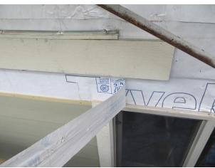
flashing integration at window head (typical).
