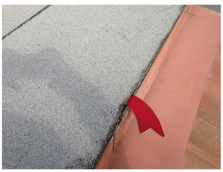
PV-01.118; 12/11/2014; B4; Roof; Membrane not sealed the drip edge
