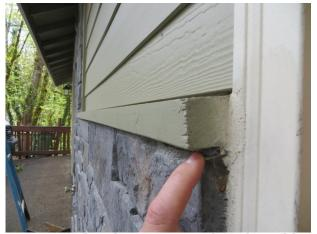
AP-02.283; Elevation Front; Overview of transition from fiber-cement siding to masonry veneer. No water table protection provided for wood trim.
