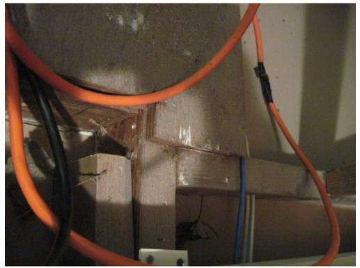
Photograph 11: Attic truss with discontinuous bottom chord
