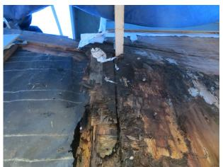
AP-01.139; Elevation Right; Damaged right elevationAP-01.141; Elevation Right; Damaged right of structure. Extensive water intrusion into building elevation of structure. Extensive water intrusion wall assembly. into building wall assembly.
