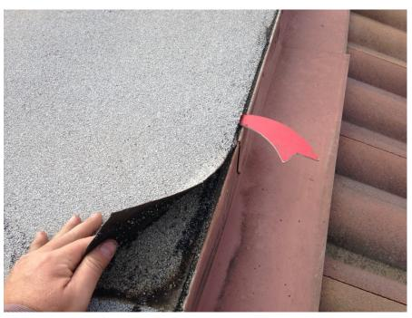
PV-01.140; 12/11/2014; B4; Roof; Membrane not sealed at drip edge
