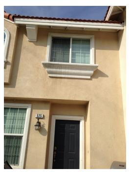
PV-01.193; 12/11/2014; B5/525; Roof - Sloped; No diverter over entry door
