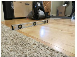
AP-02.089; Entry; High point, linear (similar to same AP-02.090; Entry; High point, linear (similar to condition in kitchen). Floor levelness does not conform to industry standards. High point is linear from entry to main living area. Separation noted at wood floors, between planks.
