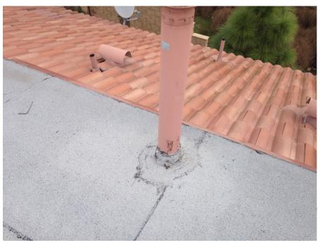
PV-01.005; 12/11/2014; B6; Roof; No storm collar at b vent
