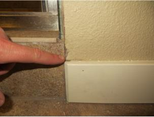
at shower enclosure frame to tile interface / inadequate sealant application and bottom of shower frame installation
