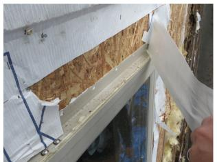
AP-02.196; Elevation Right; Improper head flashing AP-02.199; Elevation Right; Improper integration integration at window head (typical).
