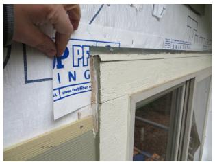
AP-02.202; Elevation Right; Improper WRB integration / Improper z-metal integration / Unprimed end cuts / reverse slope at z-metal flashing (typical condition at window heads).
