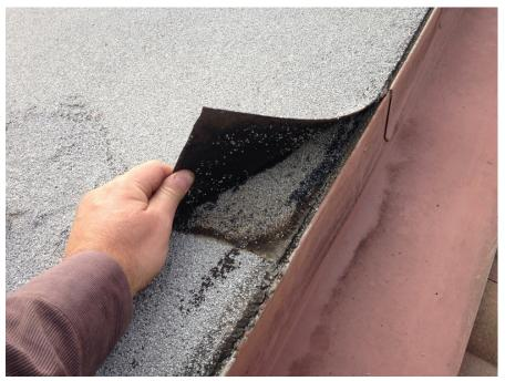
PV-01.139; 12/11/2014; B4; Roof; Membrane lap unsealed
