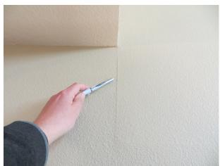
AP-02.050; Living Room; Unacceptable finishes / visible corner beads / cracks at gypsum wallboard / bowed and uneven walls
