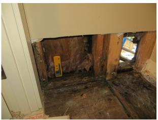
AP-01.037; Bedroom 4; Damage present at floor assembly. Organic growth present at interior of structure. Active water intrusion event. MC readings at 90% +/-.
