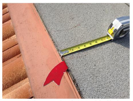
PV-01.171; 12/11/2014; B5; Roof; Membrane not sealed at drip edge
