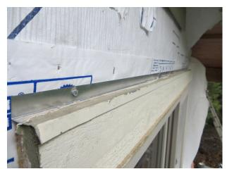
AP-02.200; Elevation Right; Reverse sloped z-metal AP-02.202; Elevation Right; Improper WRB flashing (typical).
