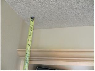
AP-02.109; Office; Office ceiling uneven, exceeding AP-02.111; Office; Office ceiling uneven, industry standards and tolerances. Cabinets noted toexceeding industry standards and tolerances. be level.
