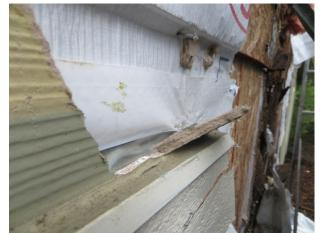
metal flashing components / Fiber cement siding sealed to metal flashing / No weep provisions
