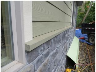
AP-02.279; Elevation Front; Improper protection of exposed water table at product transition.
