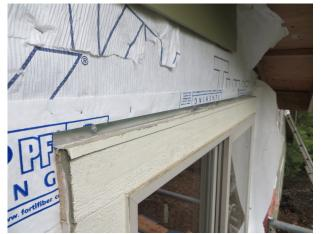
of metal flashing components / Fiber cement siding sealed to metal flashing / No weep provisions
