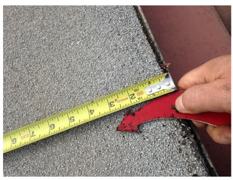
PV-01.144; 12/11/2014; B4; Roof; Membrane not sealed at drip edge
