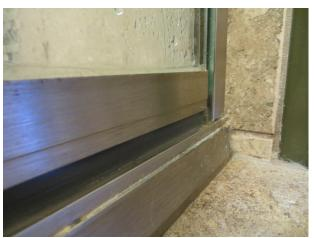
AP-02.164; Master Bath; Water reported leaking at shower enclosure frame to tile interface / inadequate sealant application and bottom of shower frame installation
