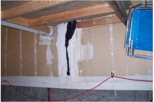
PF 01.327 PF 01- 327.jpg Garage: unit C garage - water damage at ceiling and walls. Lots of water per owner.
