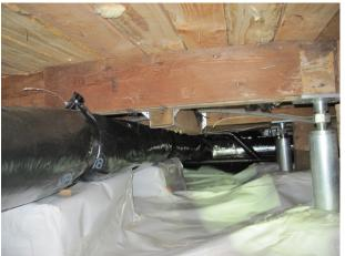
Miller Consulting Engineers-030; Uneven floor support beams. Floor jacks creating uplift, transferring through structure.
