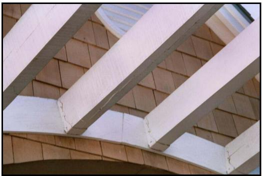
PF 02-12-036 jpg Trellis without flashing. Curved plywood ledger applied over shingles. No flashing at decorative vent above.
