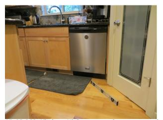
continuous from pantry to across kitchen towards refrigerator. High spot is very linear. Floor levelness towards refrigerator. High spot is very linear. Floor out of industry tolerances. Slight separation (gaps) levelness out of industry tolerances. Slight at wood flooring.
