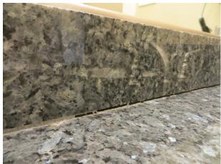
AP-02.172; Bath #2; Excessive settlement at countertop backsplash interface with horizontal surface / missing and voids at sealants
