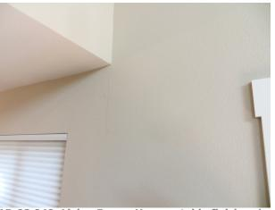
AP-02.049; Living Room; Unacceptable finishes / / bowed and uneven walls / Excessive movement at entry area
