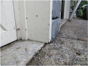
AP-02.326; Elevation Front; Inadequate clearances AP-02.338; Elevation Left; Inadequate and at product transition. Wood trim (garage jambs) in unsealed metal flashing laps. contact with concrete.
