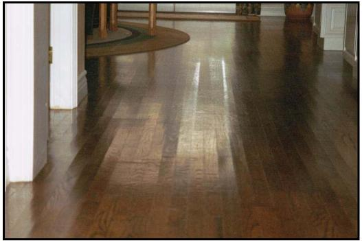
PF 04-18-090 jpg Flooring is cupped / lifting at edges across width of planks, especially between kitchen and pantry.
