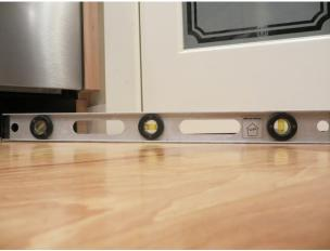
AP-02.069; Kitchen; High spot noted at pantry, and AP-02.070; Kitchen; High spot noted at pantry, and continuous from pantry to across kitchen separation (gaps) at wood flooring.
