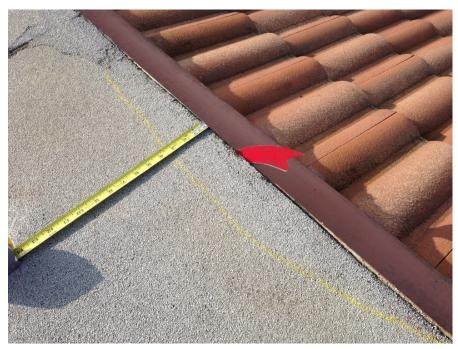
PV-01.186; 12/11/2014; B5; Roof; Membrane not sealed to drip edge at left
