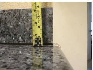
AP-02.176; Bath #2; Significant movement of granite counter-top at upstairs bathroom. Bathroom is located in the proximity of the entry.
