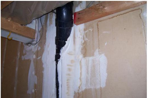
PF 01.328 PF 01-328.jpg Garage: unit C garage - water damage at ceiling and walls. Lots of water per owner.
