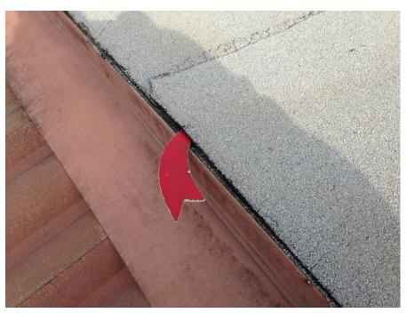
PV-01.087; 12/11/2014; B7; Roof; Membrane not sealed it drip edge
