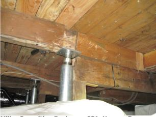
Miller Consulting Engineers-031; Uneven floor support beams. Floor jacks creating uplift, transferring through structure.
