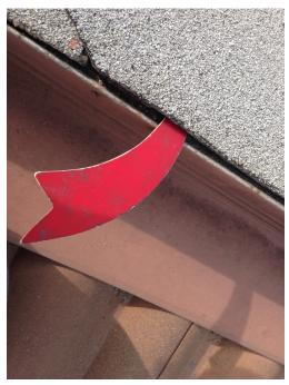
PV-01.082; 12/11/2014; B7; Roof; Membrane not sealed to flashing
