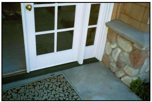
PF 06-14-014.jpg Exterior at French doors. Casing buried by masonry. Doors splitting.
