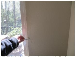
AP-02.047; Living Room; Unacceptable finishes / visible corner beads / cracks at gypsum wallboard / visible corner beads / cracks at gypsum wallboard bowed and uneven walls
