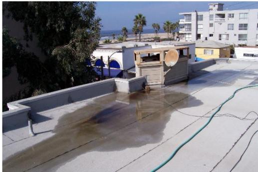
PF 01.135 PF 01- 135.jpg Roof test A: water is ponding around drain at right elevation near chimney.
