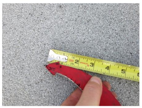
PV-01.120; 12/11/2014; B4; Roof; Membrane not sealed the drip edge
