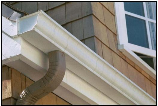
PF 01-15-015 jpg Standard gutters are being over-shot by steep sloped roof.
