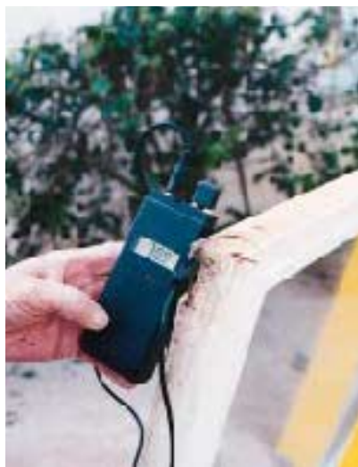
Figure 11. Wood windows should be painted on all raw wood surfaces. Otherwise, they will pick up excessive moisture (as the moisture meter reading in the photo at right shows), causing them to swell or even rot.
