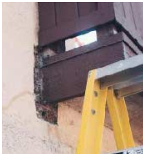
Figure 12. Framing protrusions, such as handrails (left) and cantilevered joists (right), are difficult to flash properly, inevitably leading to moisture intrusion, cracked stucco, and decay in the structure below.
