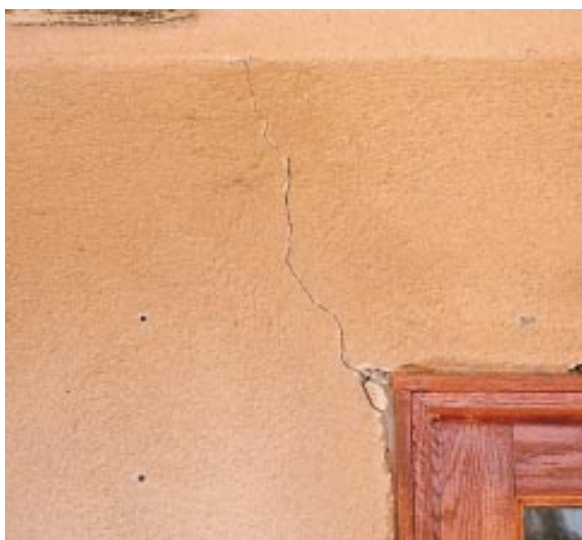
Figure 14. Stucco cracking is one of the most common customer complaints. Tight surface cracks are normal in stucco and can usually be repaired. With quality workmanship, larger cracks can be avoided.
