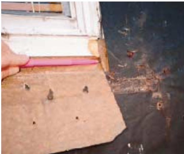
Figure 10. Here, the building paper is installed under the flashing paper at the bottom of the window, but not on the side — leaving a vulnerable corner where the flashing paper has been cut.
