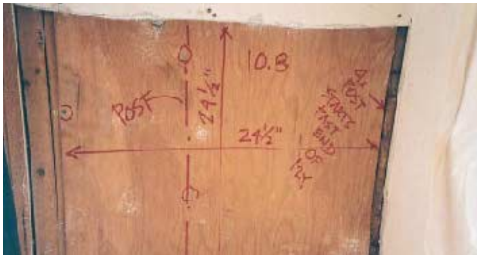
Figure 3. This shear plywood falls short of the shear wall posts on the right and left, and is attached with too few nails.
