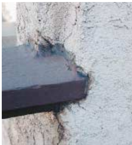
Figure 12. Framing protrusions, such as handrails (left) and cantilevered joists (right), are difficult to flash properly, inevitably leading to moisture intrusion, cracked stucco, and decay in the structure below.
