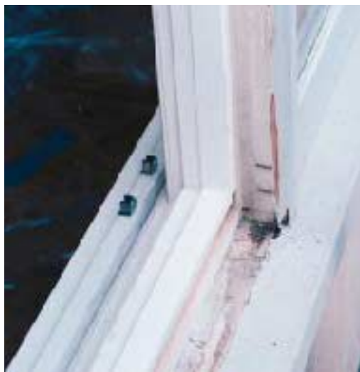
Figure 11. Wood windows should be painted on all raw wood surfaces. Otherwise, they will pick up excessive moisture (as the moisture meter reading in the photo at right shows), causing them to swell or even rot.
